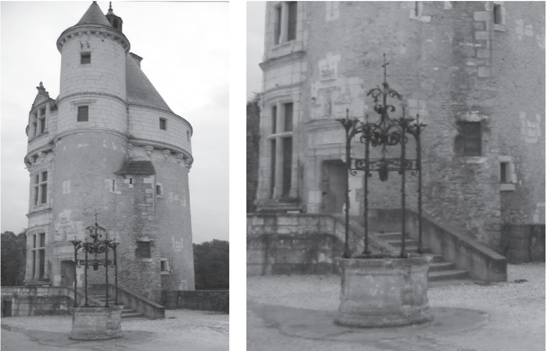
Figure 4.15 Medieval well with reel (type AV) and tower, Castle Chenonceau, Loire Valley, France. (Photo: Petri Juuti)
