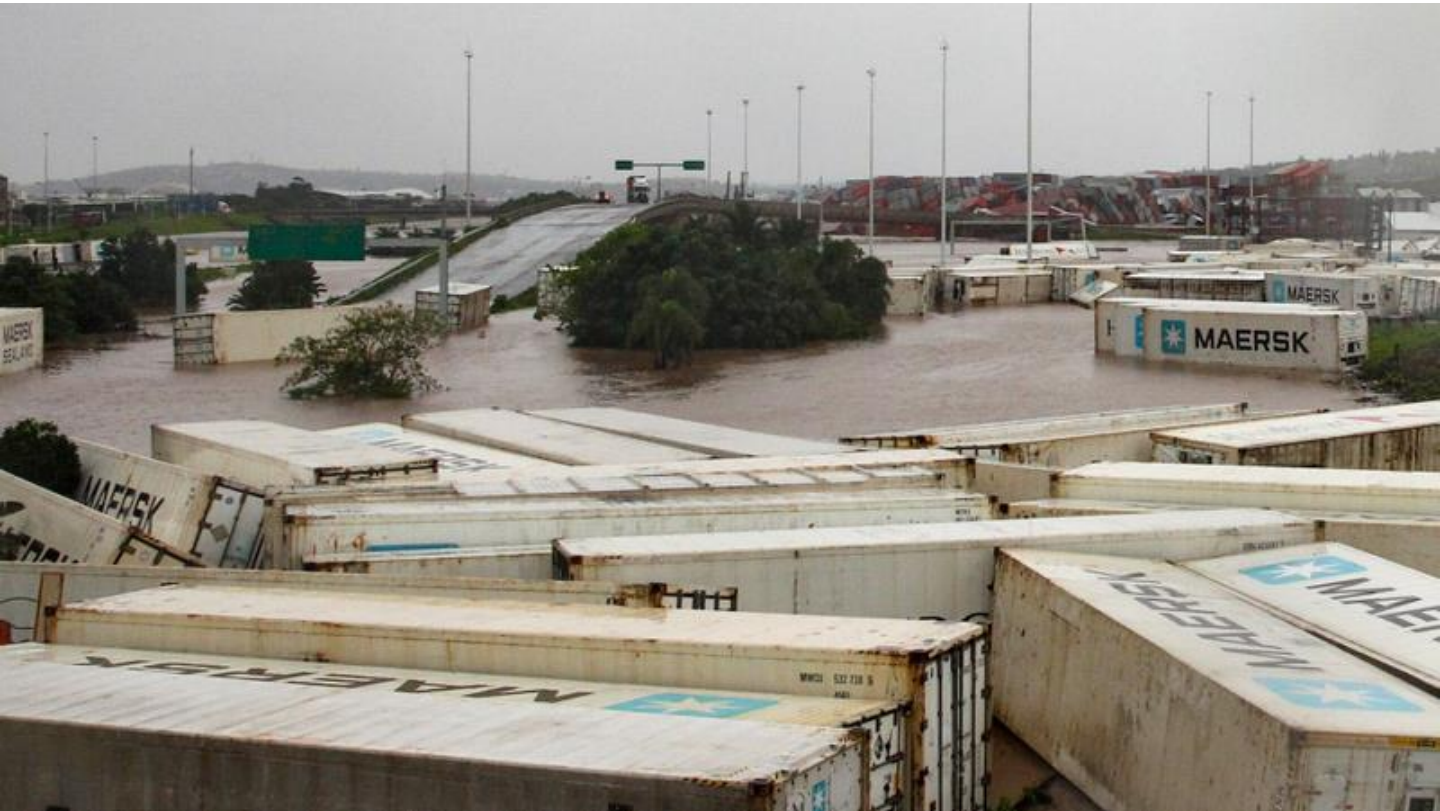
Shipping containers shifted by floods
