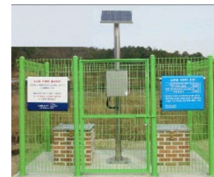
[ Groundwater monitoring well Installation ]
