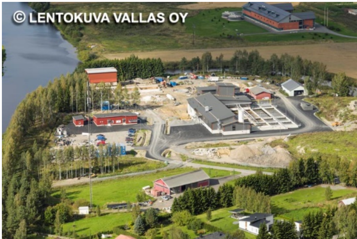
Nearly completed plant in summer 2016
