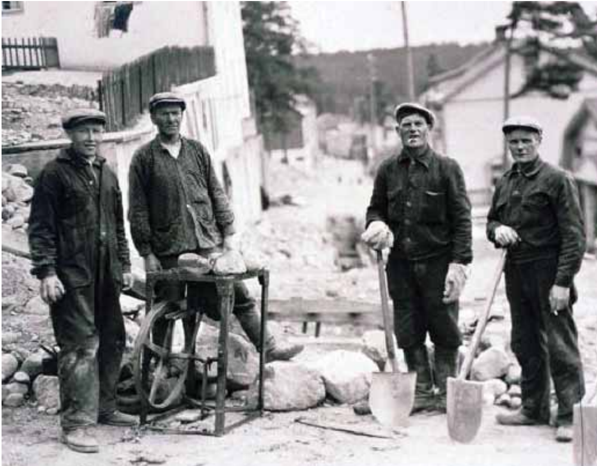
Picture N° 2. Installing the water mains.
