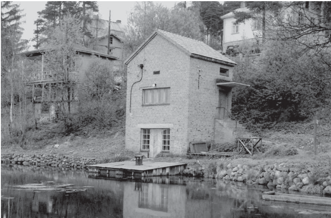
Picture N° 4. Pumping station of the Pispala water cooperative in 1952.
