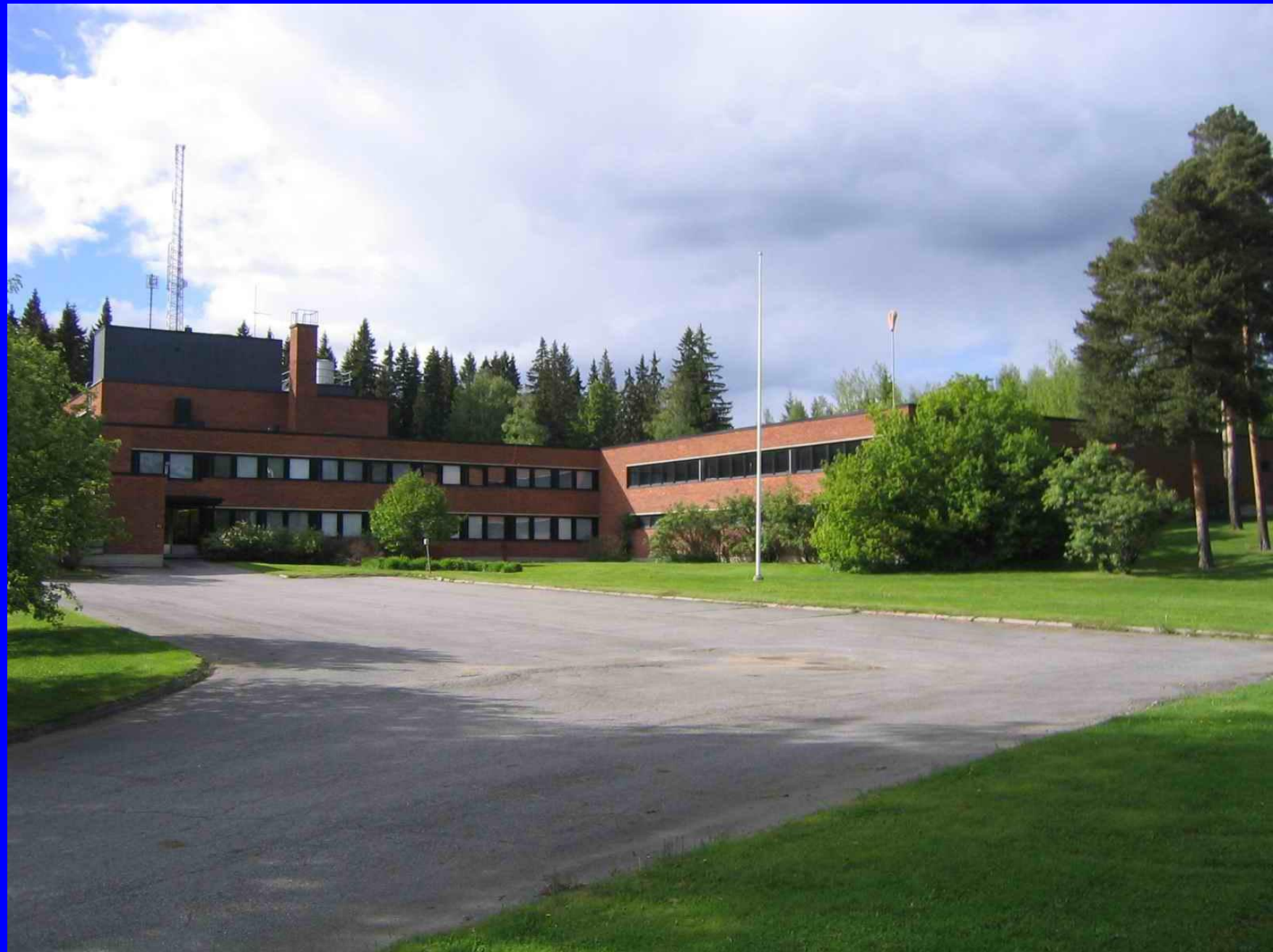
Rusko water treatment plant
